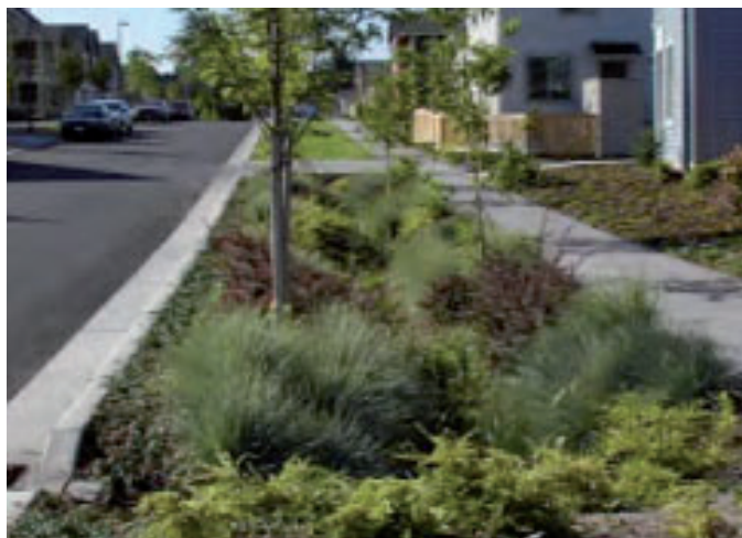
Figure 13.5: Vegetated drainage channel
